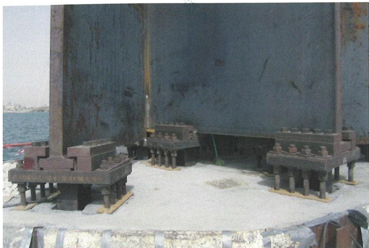
This page, top: The sculpture, 7, is erected on an artificial pier along Doha's waterfront. Photos on p. 96 courtesy of Leslie E. Robertson Associates. This page, middle: The seven plates are anchored with mechanical joints at the base.
